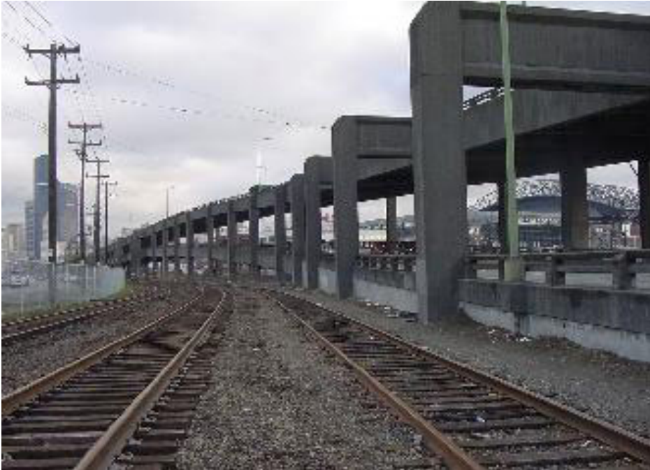
Figure 24—Photo of the Alaskan Way Viaduct, Seattle, showing location of point at which northern boundary of observed liquefaction occurred (Photo by Bray and others, 2001).
