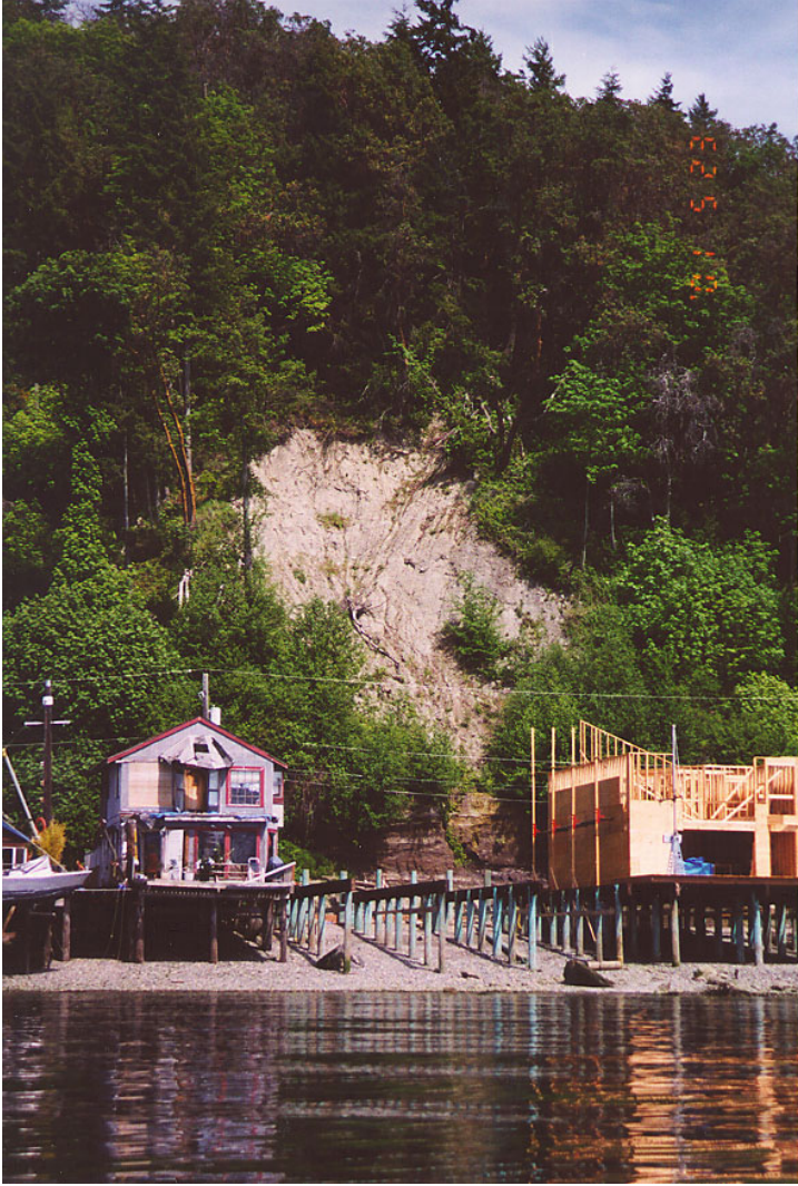
Figure 5–Salmon Beach house, destroyed by landslide. The house was damaged and then was torn down. The house under construction to the right, is being rebuilt, as it was also destroyed by the landslide (Photo taken in June, 2001 by Lynn Highland, USGS).
