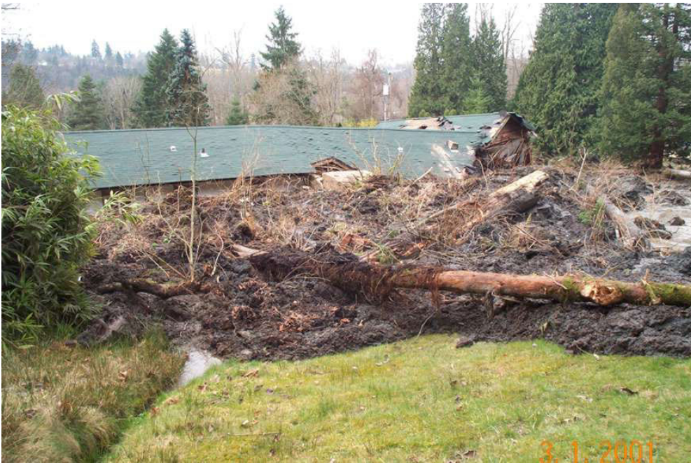
Figure11—House damaged by landslide along Cedar River—landslide deposits are at the center of the photo (Photo courtesy of King County, Washington, February, 2001).
