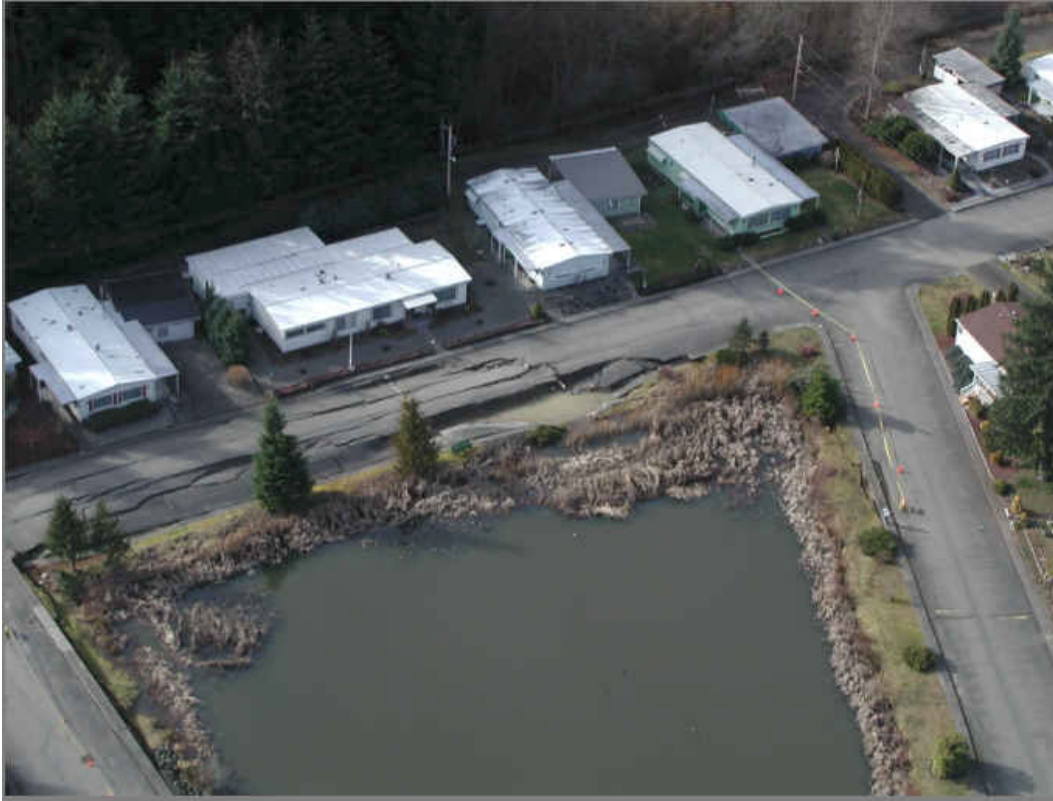
Figure 19—Aerial view of the lateral spread that occurred along a perimeter road of Sunset Lake, near Tumwater. The street affected by the flow is roughly aligned north-south where north is toward the bottom right corner of the photo (Photo from Bray and others, 2001).
